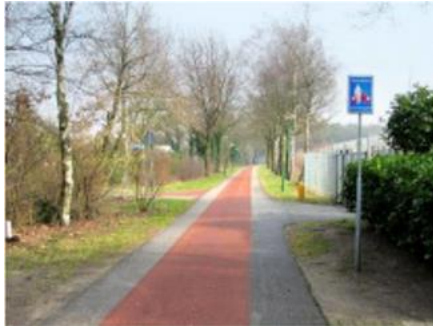
Figure 2: Cycle Street Netherlands
