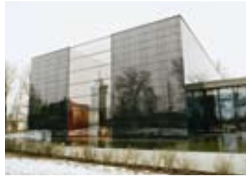
35 St. Francis Parish Buildings Wels / OÖ
