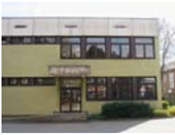
The 1970s building
